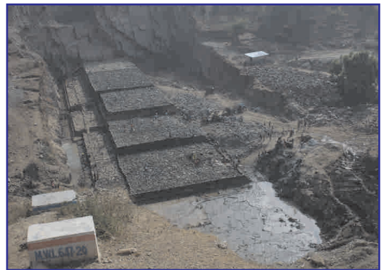
Akodara Dam (Under Construction)
